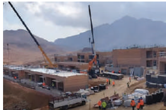
Trojena Base Camp – Neom
