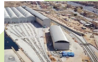
Riyadh Metro, East & South Depot Riyadh
