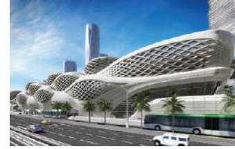
Riyadh Metro - Line 1 King Abdullah Financial District Parcel Station
